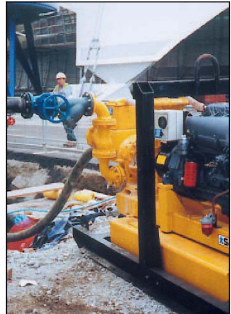
Pressure Test & Flush
